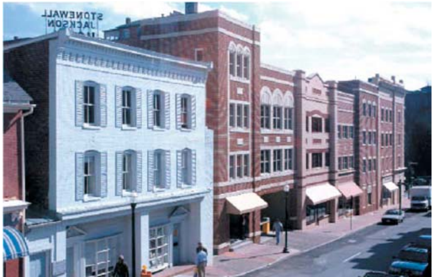
Retail space is located on the street level of the west elevation, hiding the fact that there's an enormous parking garage in the building. The modulated structure gives the impression of a series of several smaller buildings, rather than one large space. (Photo by Jason Hottel Photography)
