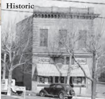
Located on a prominent corner in Altavista, the work on this building included the reconstruction of missing cornices and windows that replicate the original elements. New signs and awnings were also added. The historic photograph was used to guide the design.
