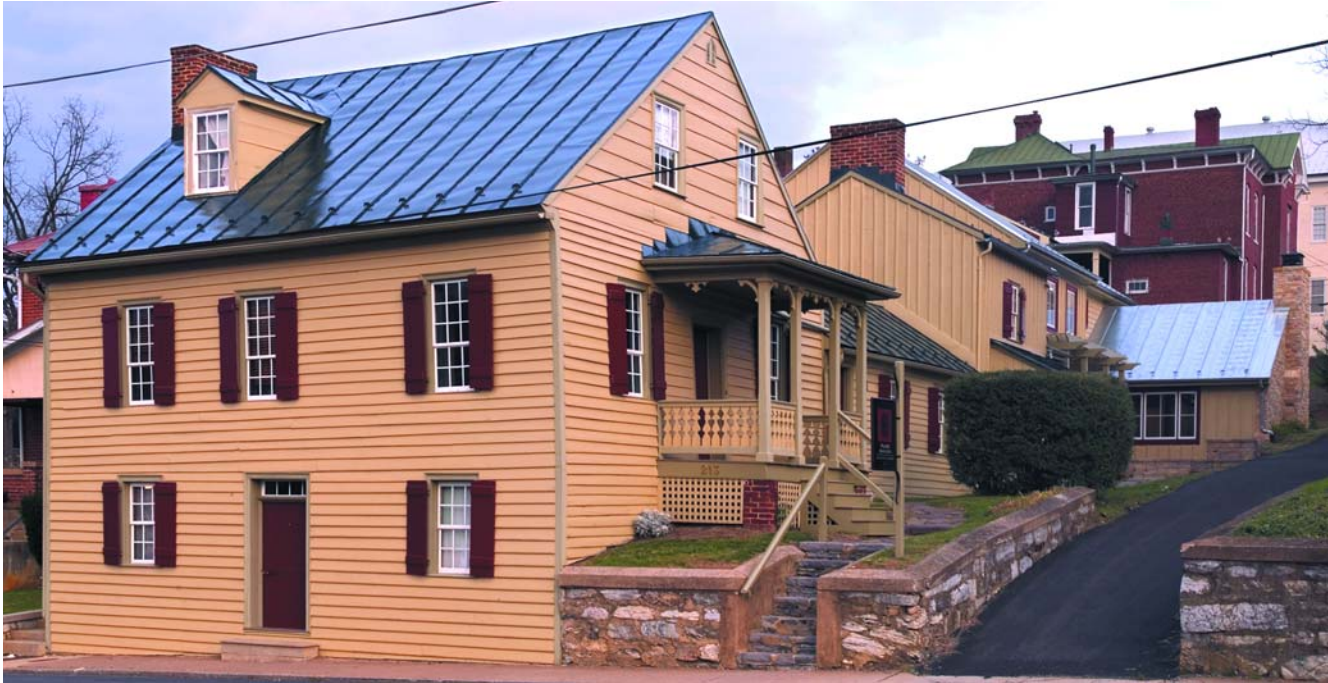
Fig. 1. March of buildings continues with completion of addition. Original log structure at front, two 19th-century additions next, compound 21st-century timber frame last, terminating in masonry chimney at far right, the end of the conference room.
