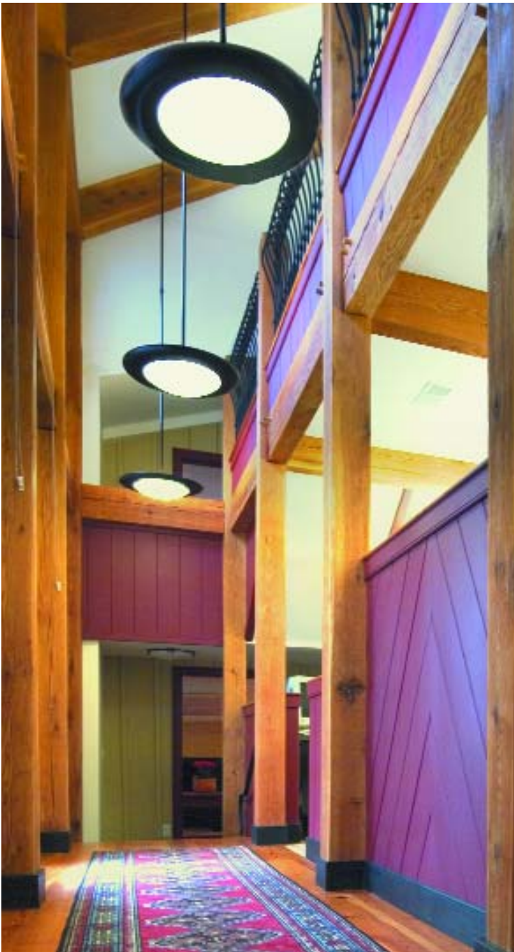
Fig. 5. Two-story light well has double-height south-facing windows. Curved iron balusters were forged by local blacksmith.
